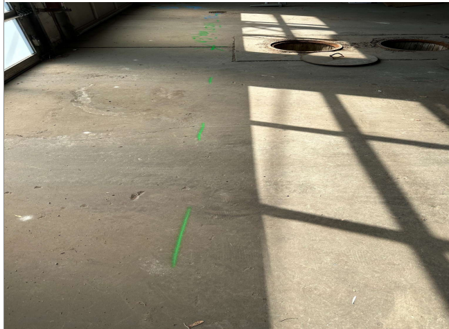
Storm Pipe - Unit 9 Alignment (Green markings)
