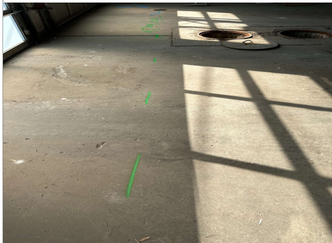
Storm Pipe - Unit 9 Alignment (Green markings)
